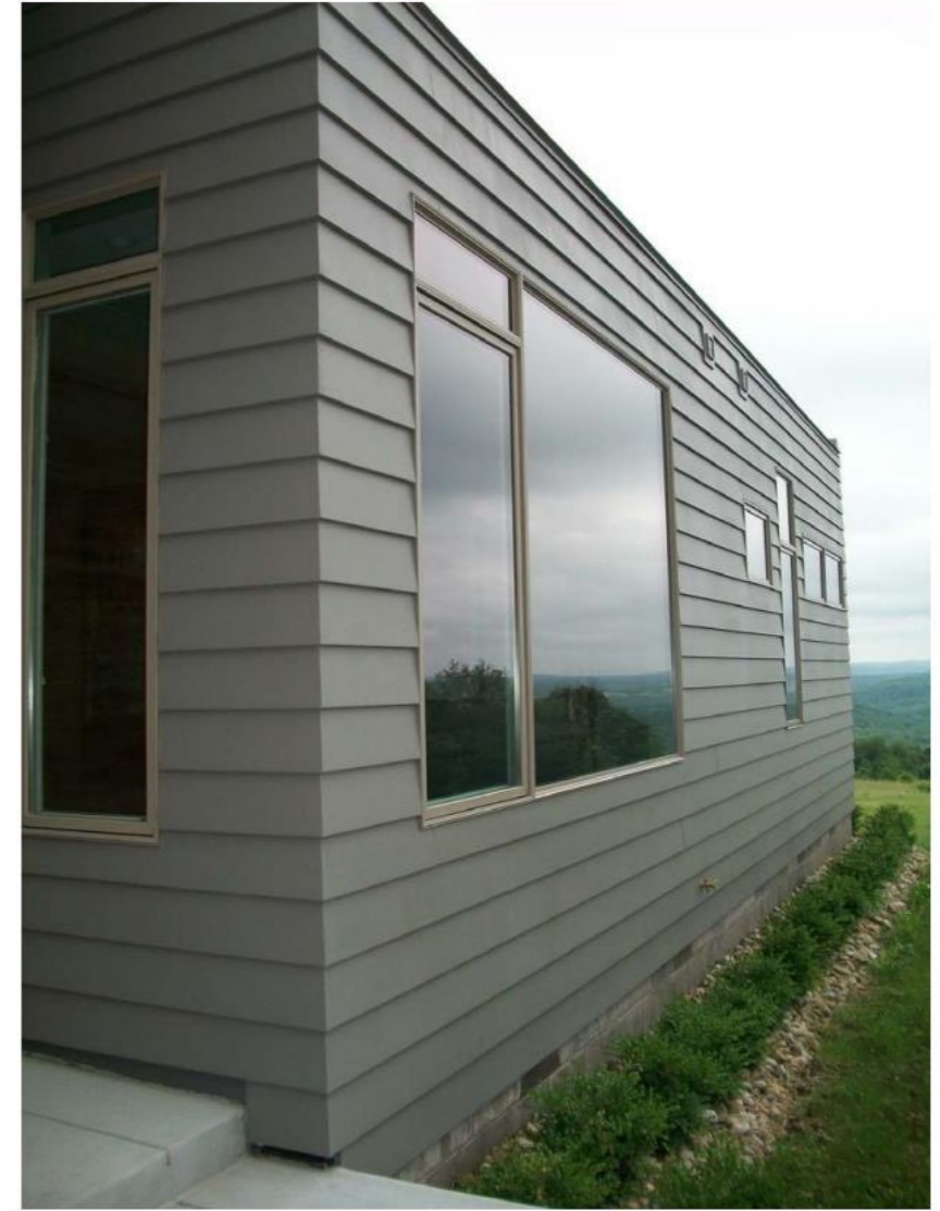
LAP SIDING - MITERED CORNER
