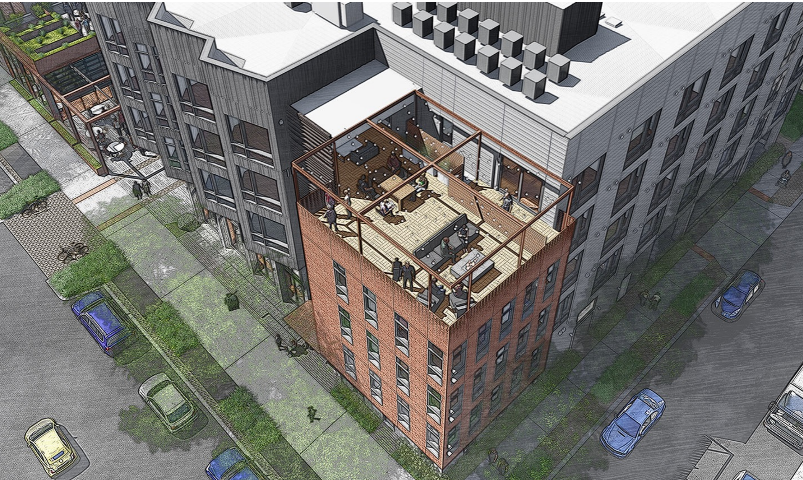
C. Walls Facing Roof Terrace
