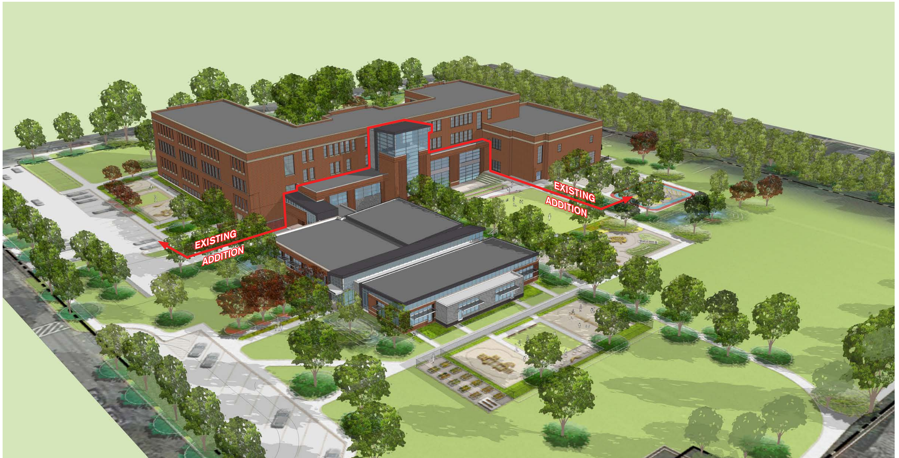
OVERALL VIEW LOOKING NORTH
