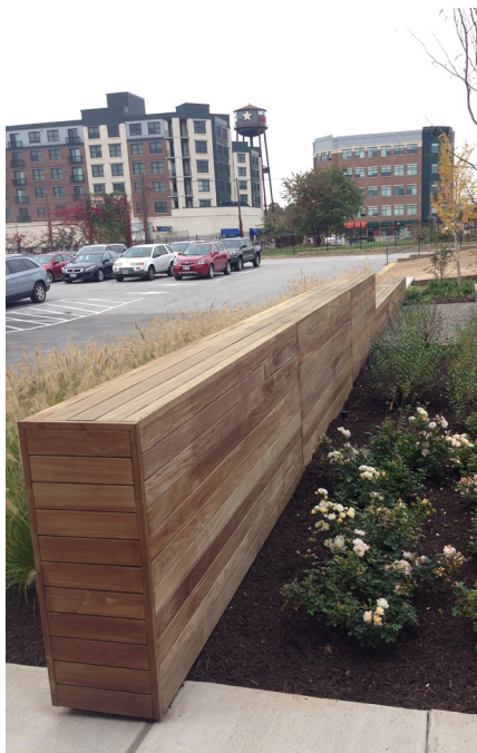
IPE-CLAD CONCRETE WALLS
