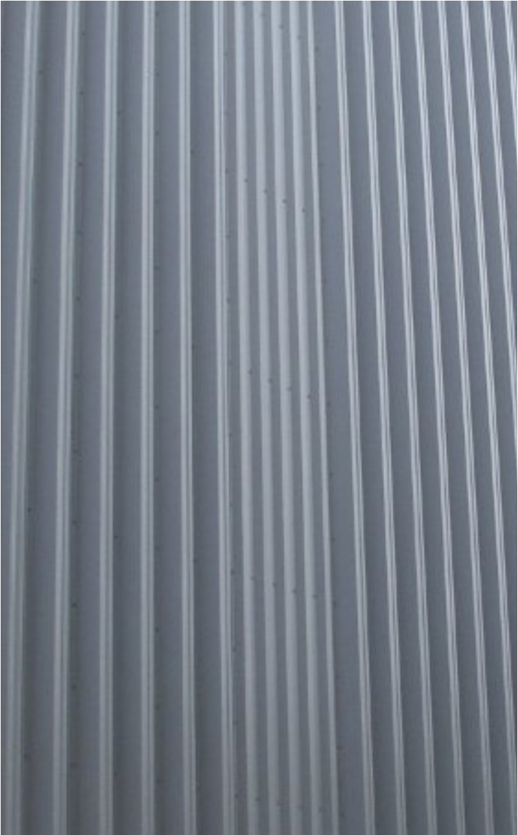
CORRUGATED METAL PANELS
