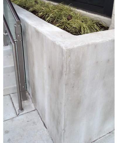
RUBBED CONCRETE WALLS
