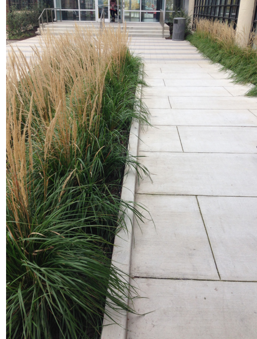
DECORATIVE SCORED CONCRETE PAVEMENT
