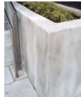
RUBBED CONCRETE WALLS
