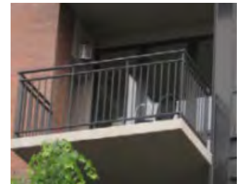
PAINTED METAL PICKET BALCONY
