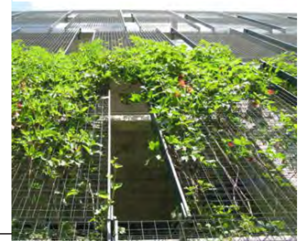
ARCHITECTURAL METAL MESH MID-FILL w/ PLANT WALL
