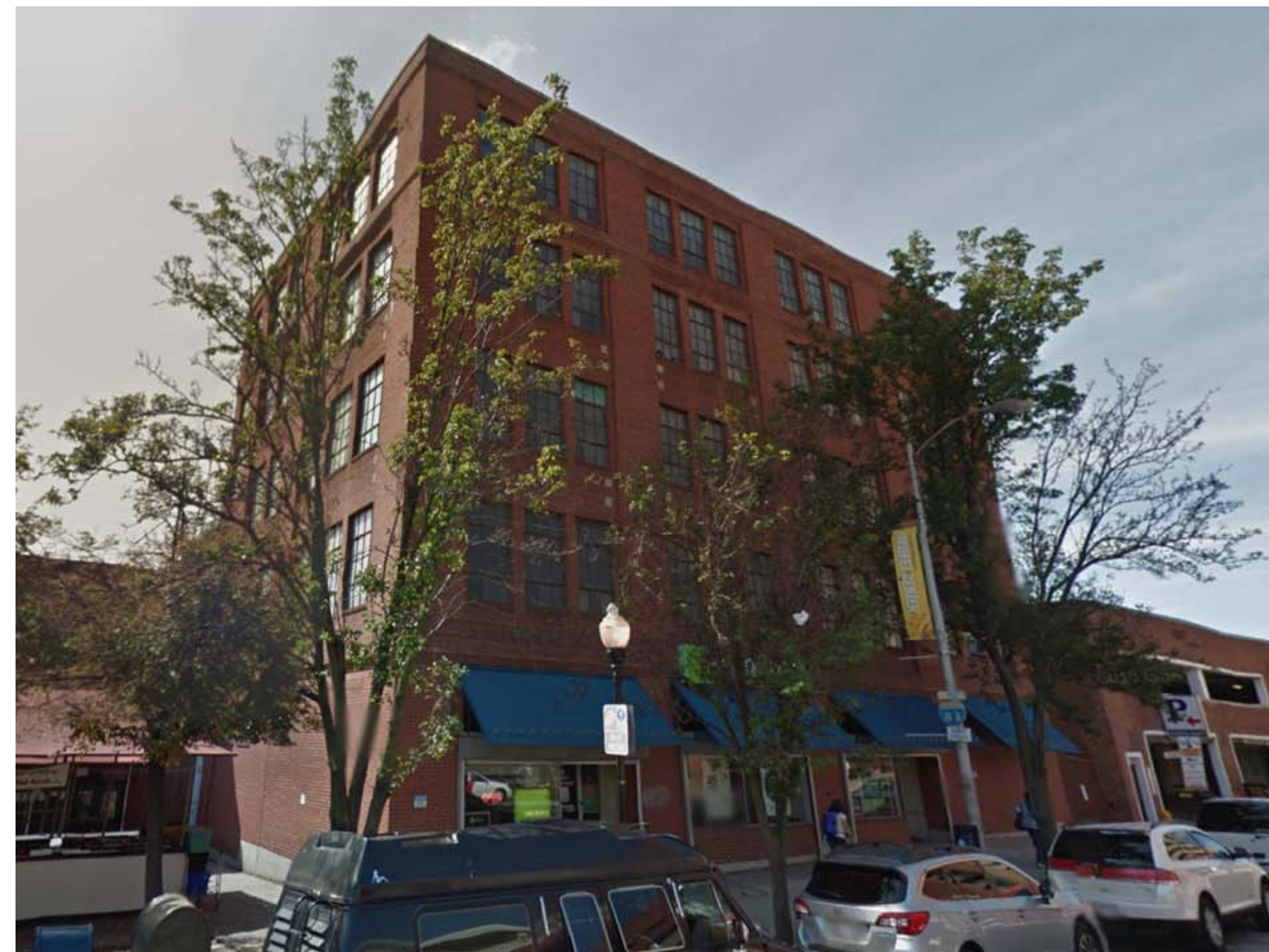
Greater Context: Masonry Loft Buildings
