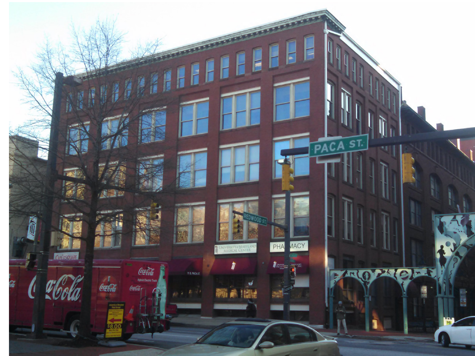
Greater Context: Masonry Loft Buildings
