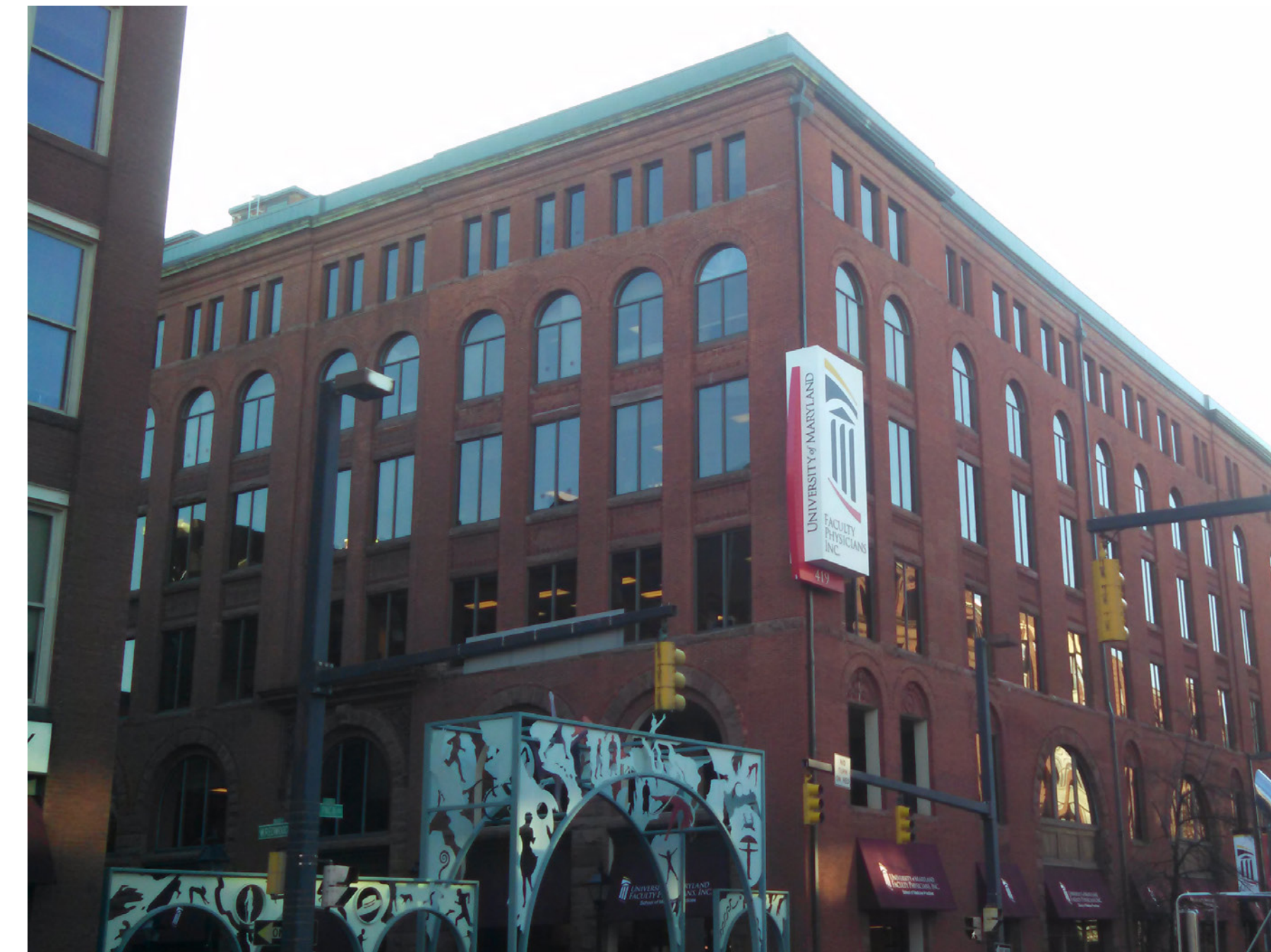
Greater Context: Masonry Loft Buildings
