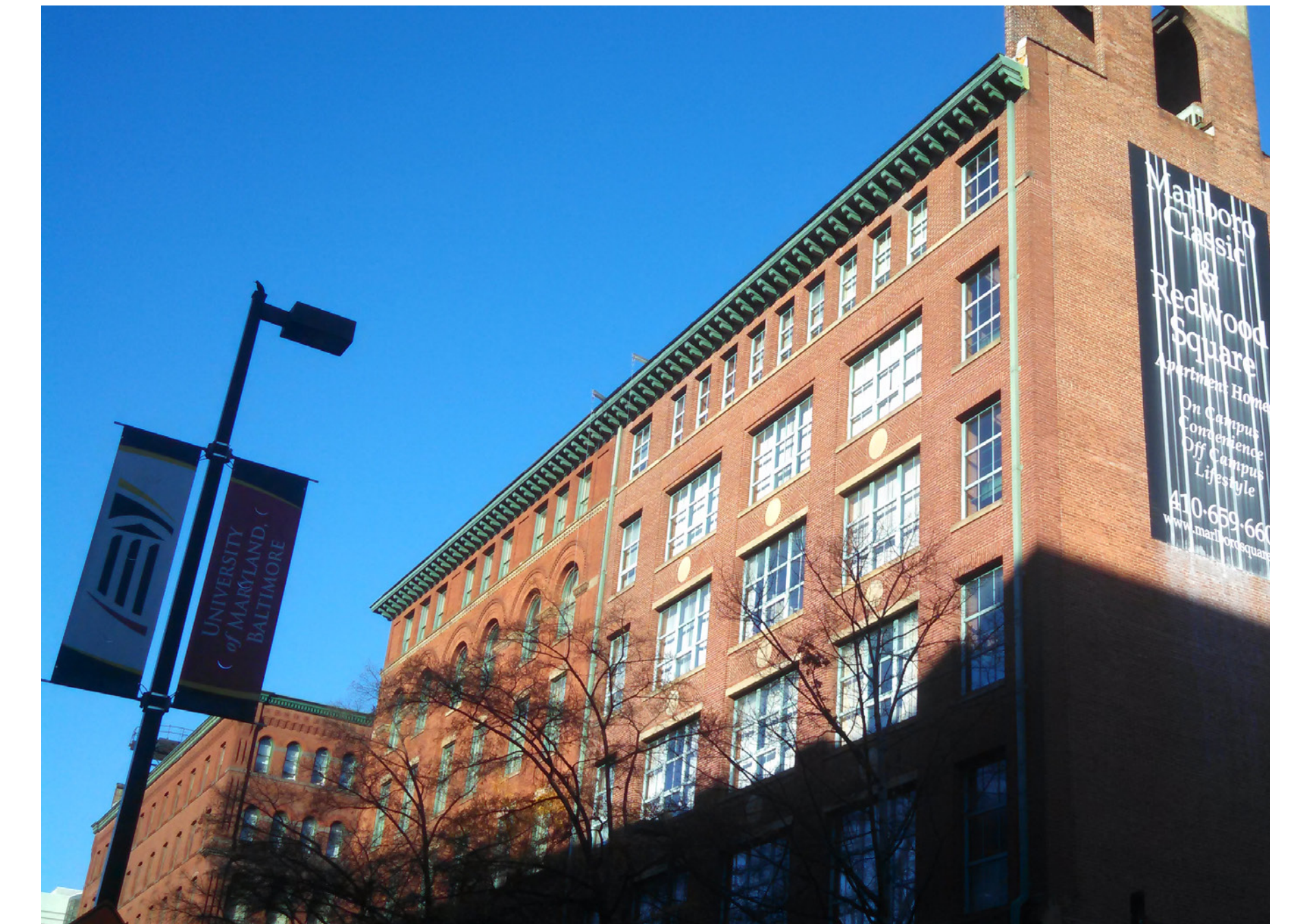
Greater Context: Masonry Loft Buildings
