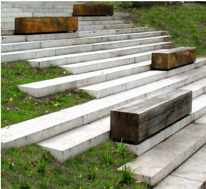
STAIRS: LIMESTONE AND WOOD BENCHES
