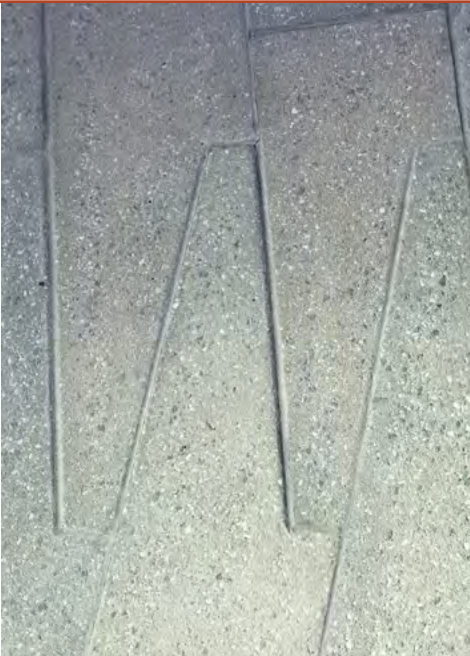
DINING TERRACE: COLORED CONCRETE WITH EXPOSED AGGREGATE
