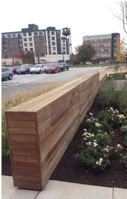
IPE-CLAD CONCRETE WALLS
