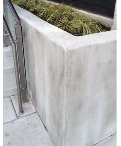
RUBBED CONCRETE WALLS
