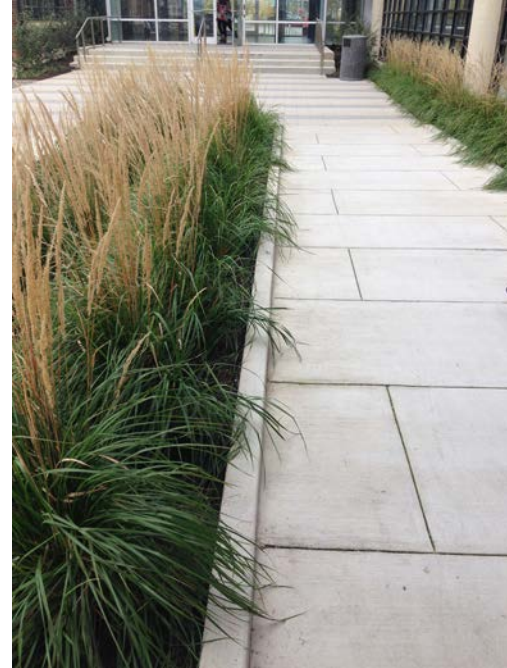
DECORATIVE SCORED CONCRETE PAVEMENT
