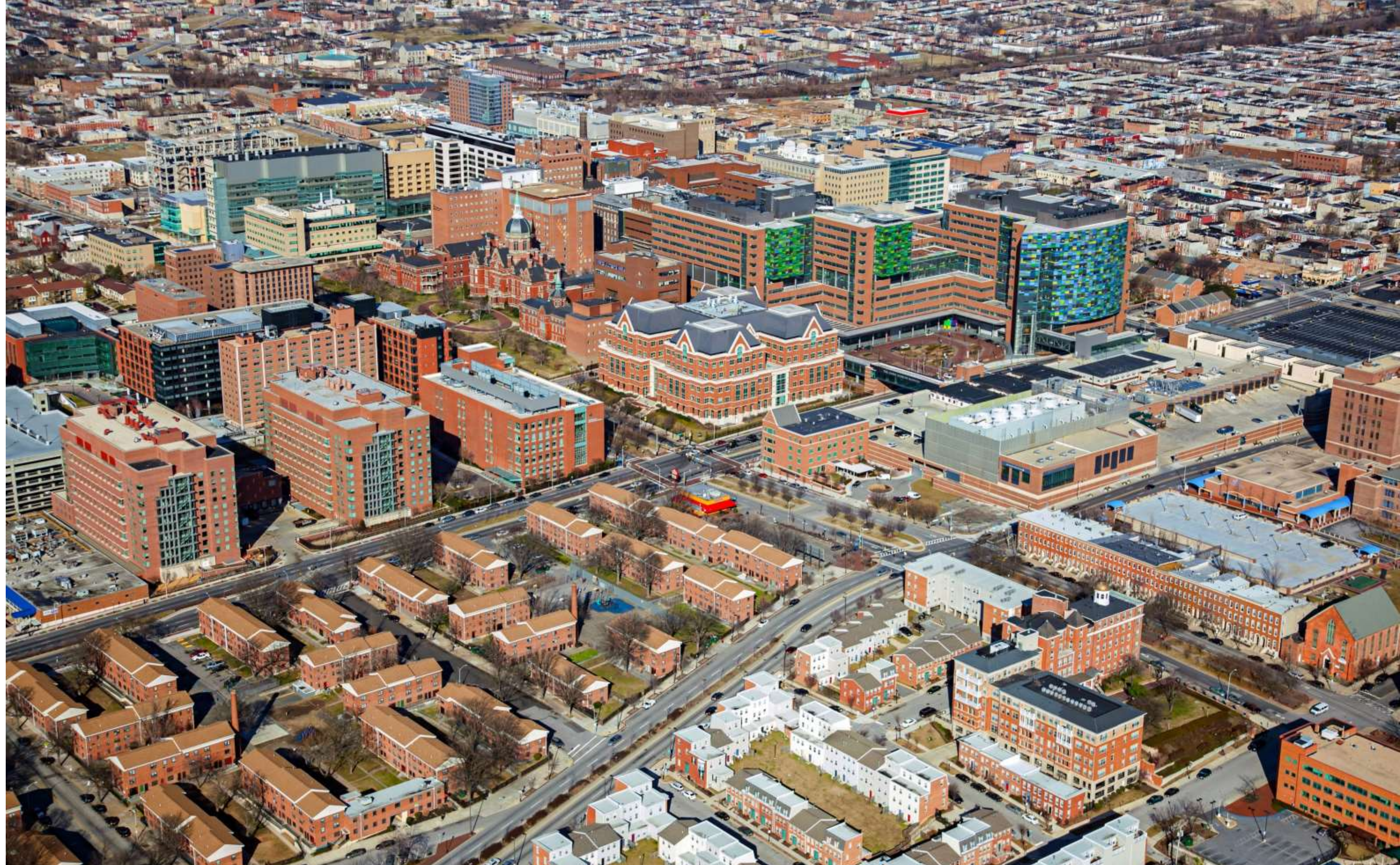
Aerial view looking northeast at Johns Hopkins Hospital
