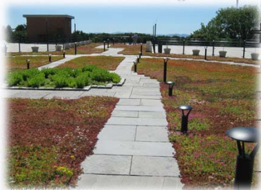
PLAZA PAVERS: LARGE FORMAT PORCELAIN PAVERS ON PEDESTALS FLUSH WITH GREEN ROOF SURFACE
