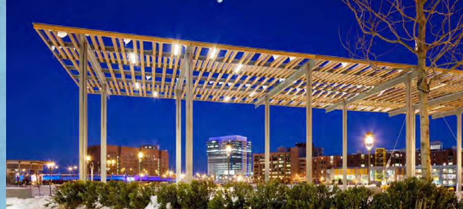
SHADE STRUCTURE: WOOD & STAINLESS STEEL
