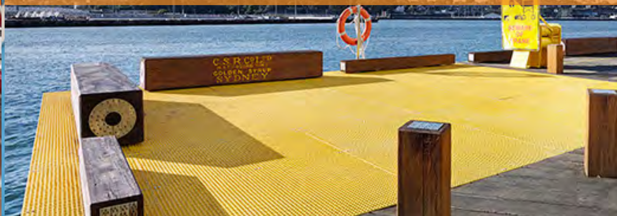
KAYAK LANDING: FIBERGLASS DECKING
