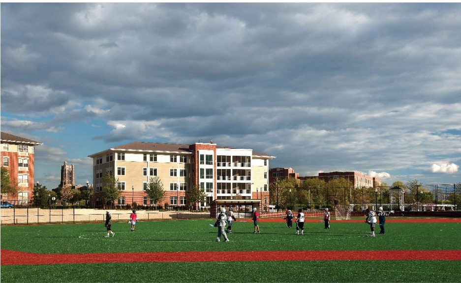
View from field looking North at Stadium Place
