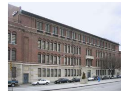
Existing campus building
