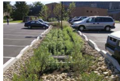
Adding permeable planting beds to surface parking provides a creative solutions for storm water collection
