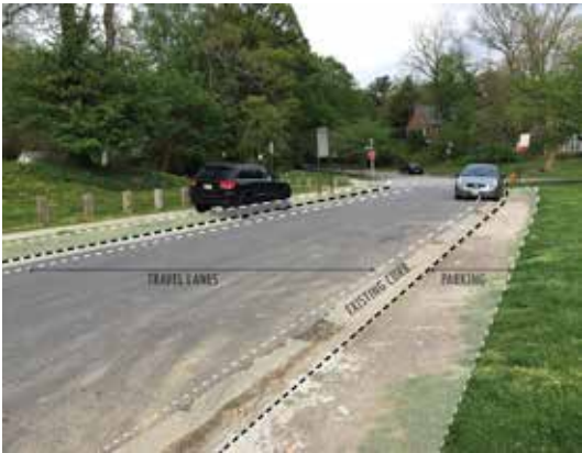
Example of parallel parking on permeable pavers
