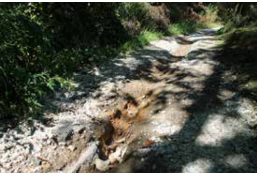
The condition of the walking path is deteriorating in some areas
