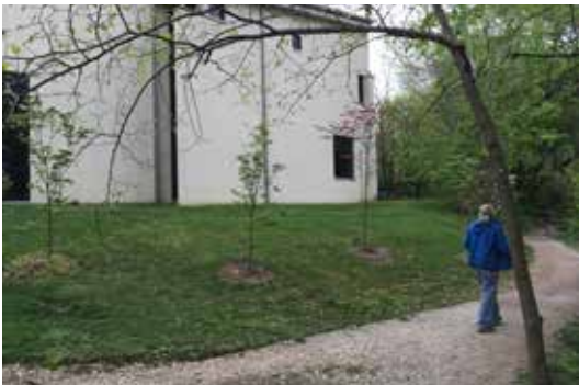
The Bolton Street Synagogue building
