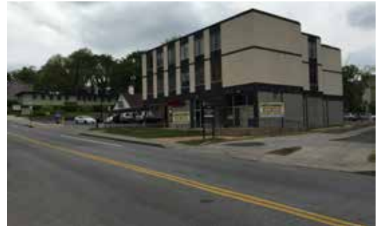
Existing condition at the Professional Building
