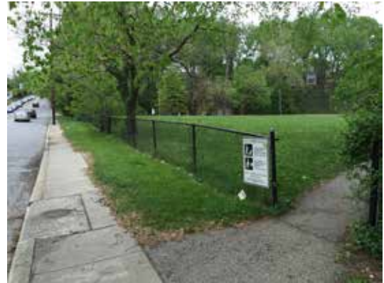
Existing condition along south side of Cold Spring Lane
