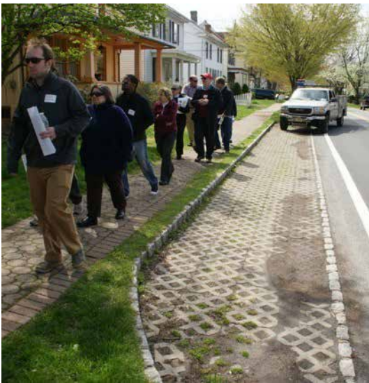
Example of parallel parking on permeable pavers
