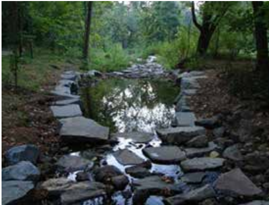
Stony Run stream restoration project. (Source: Department of Public Works)
