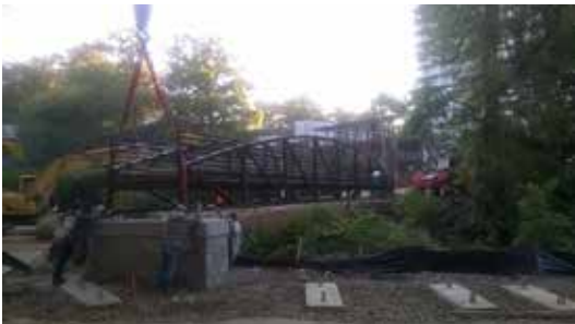
Pedestrian bridge construction
