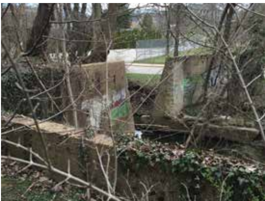
Remnant walls at the northern section
