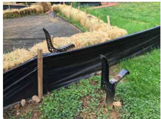
Benches removed for the bridge construction
