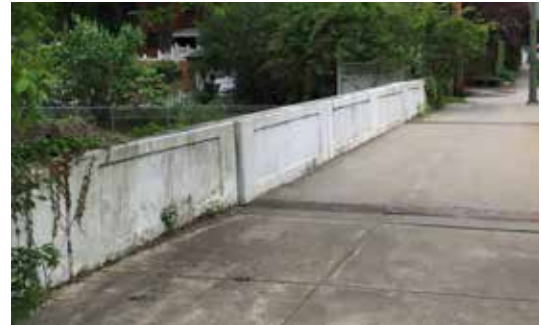
Bridge abutments provide an opportunity for public art
