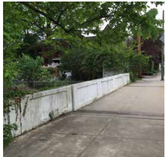
Bridge abutment along Cold Spring Lane, potential for public art
