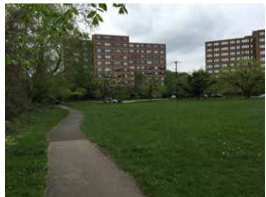
Linkwood Park, path along the western edge
