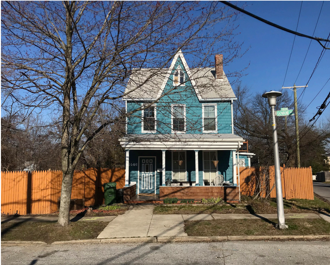
Photo 4. Distinctive wood shingle frame house at 5601 Govane Avenue in Mid-Govans built in 1870, 2018 March 12.
