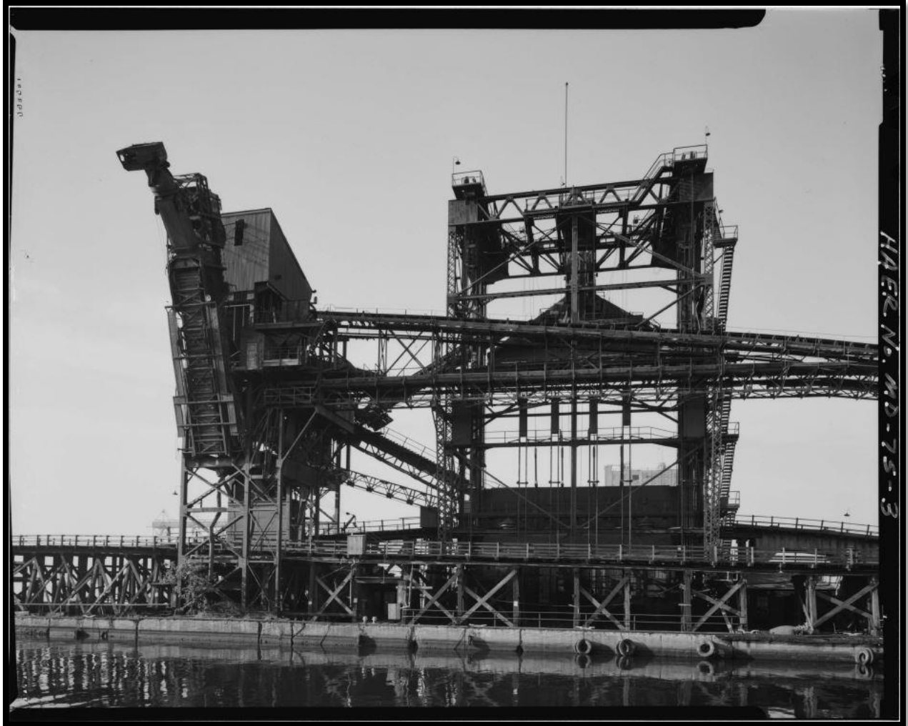
Port Covington coal pier. Credit: Library of Congress, Prints & Photographs Division, HAER, HAER MD,4-BALT,190—3
