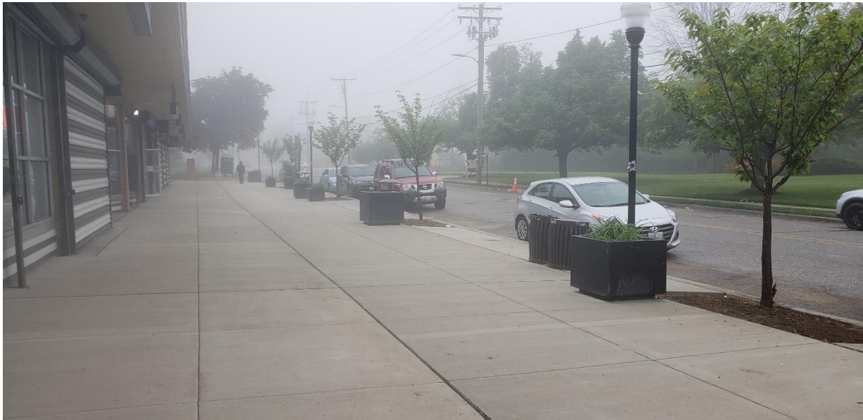
Sidewalk installation completed May 2019.
