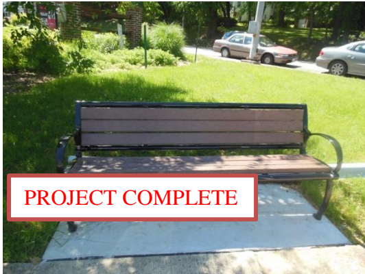
Installation of Benches in the Business District was completed March 2016.
