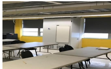
Northern Bldg. #402 – AC project complete
