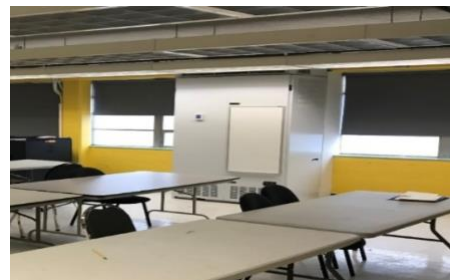
AC project complete at Northern HS Bldg.
