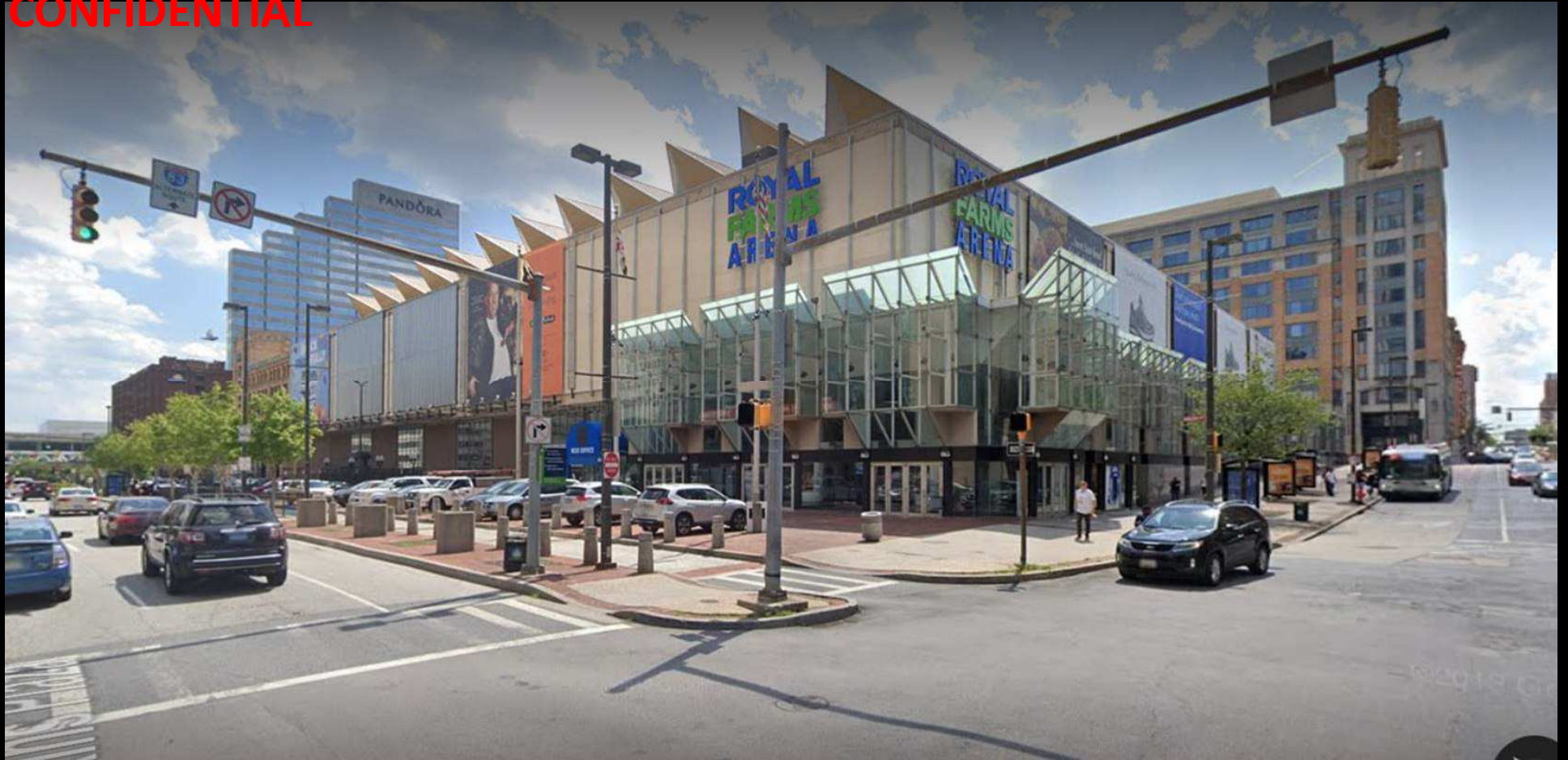
Existing Exterior Hopkins Plaza and Baltimore St W
