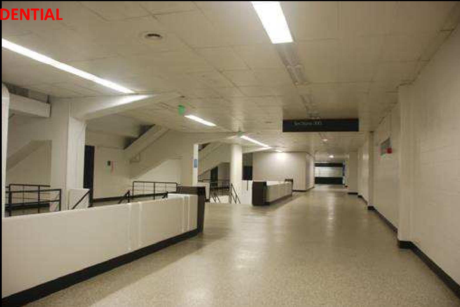
EXISTING LEVEL 4 NORTH CONCOURSE
