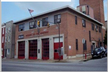
Fire station renovations
