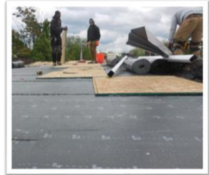
Vacant Property Roof Stabilization
