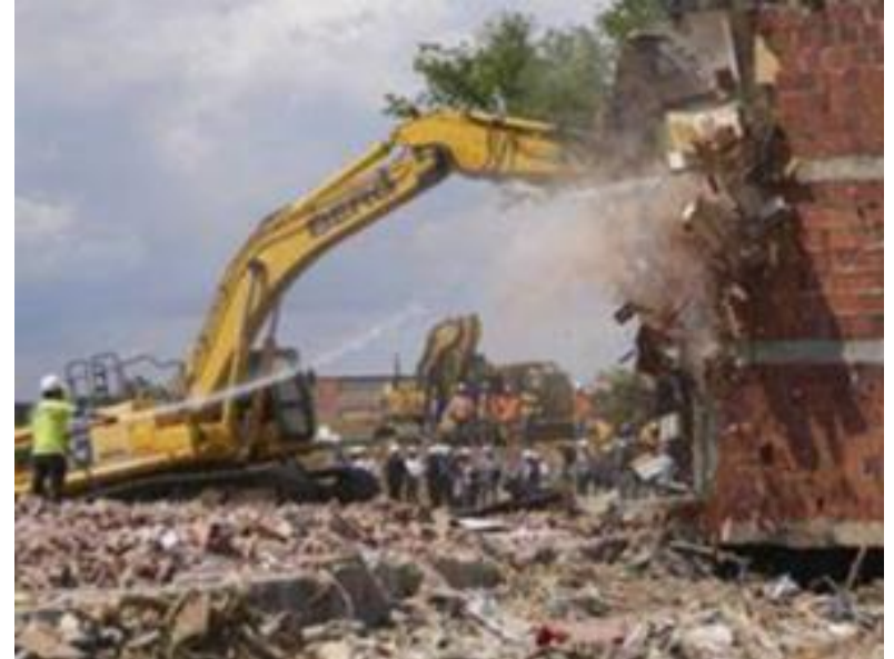
Demolition at Perkins
