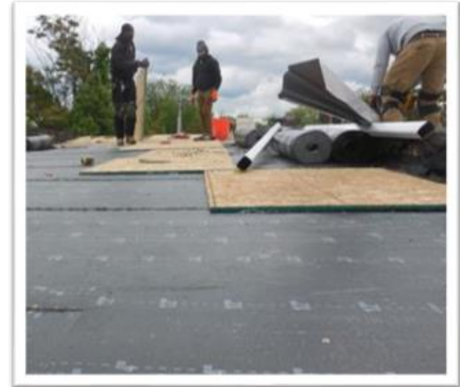
Vacant Property Roof Stabilization
