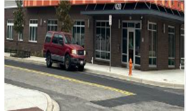
New Sidewalk and Road Infrastructure at Somerset
