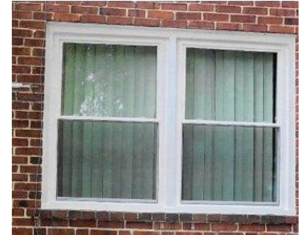
New window and exterior basement Bilco door installation
