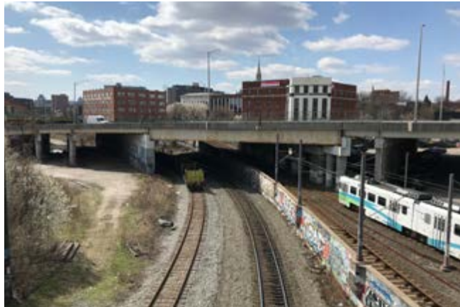
MTA Light RailLink under Interstate 83.
