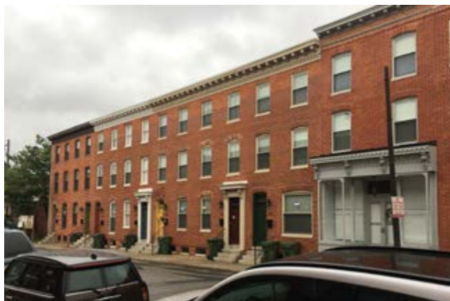
Rehabilitated rowhomes that received the CHAP Tax Credit at 1200 block of Gay Street.
