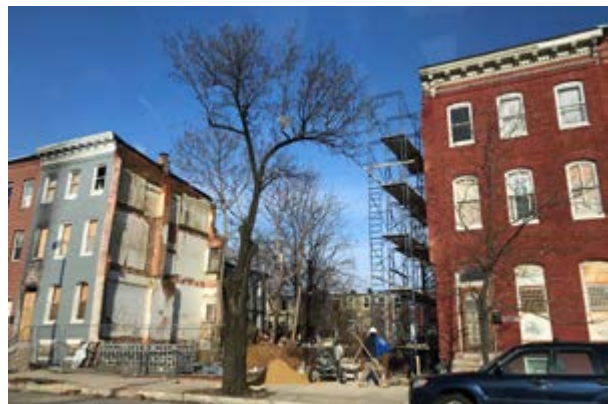
Demolition site next to a vacant rowhouse, northwest corner of Wilkens Ave. and Monroe St.
