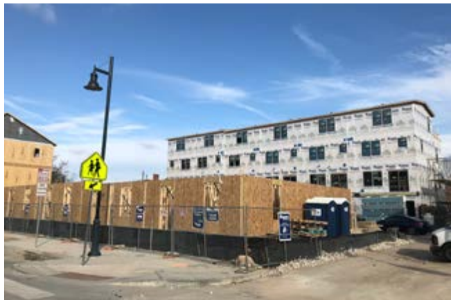
Construction of new residential housing.
