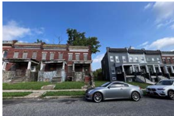
Vacant and renovated houses in Greenspring.
