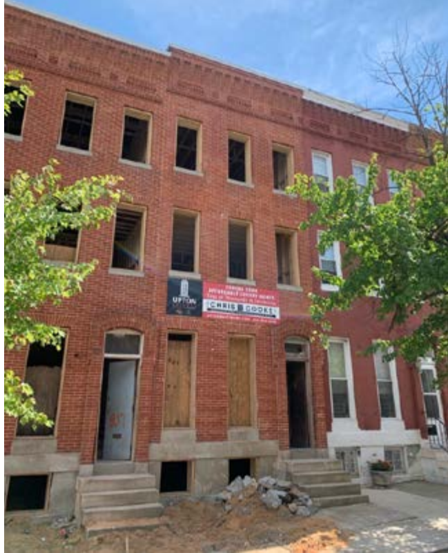
Renovation underway in Upton.
