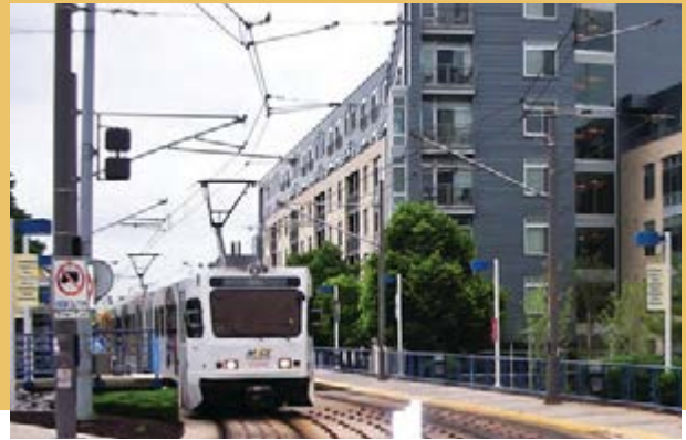
The Fitzgerald apartment building next to the MTA Light RailLink Mt. Royal / MICA Station.
