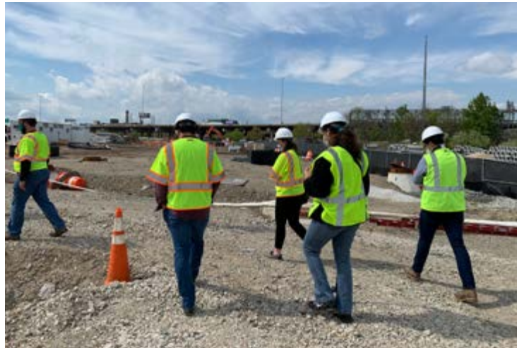
A construction site in South Baltimore.
