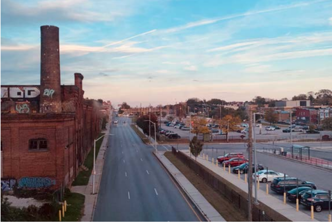
The American Ice Building adjacent to the West Baltimore MARC Station has been the subject of TOD proposals in past years.
