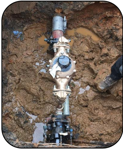
AMI/R new meter install
