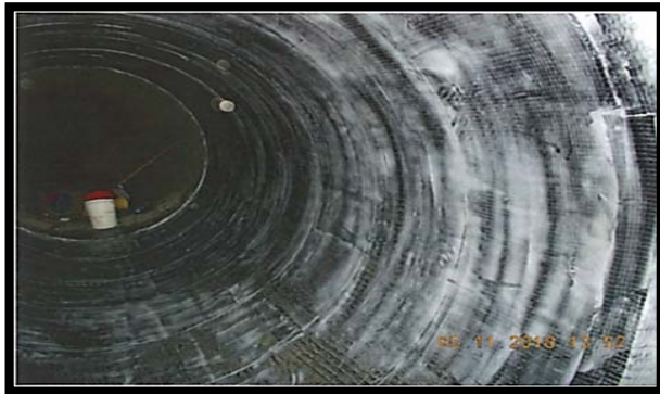
Proactive Internal Carbon-Fiber Repair of 84" PCCP
