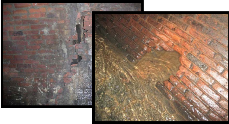
Missing mortar and bricks
