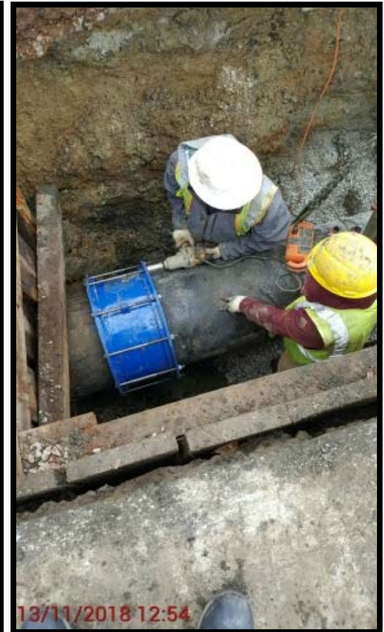
DIP water main replacement
