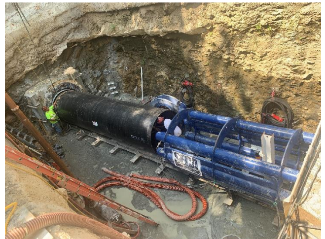
SC-910: Microtunneling under Perring Parkway
