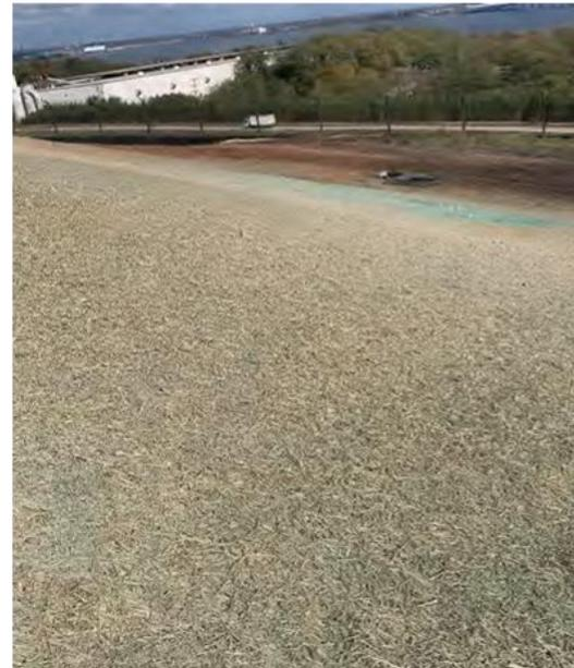
QRL cell 6 area (upper E slope) graded and hydro-seeded for soil stabilization as per MDE compliance requirement.
