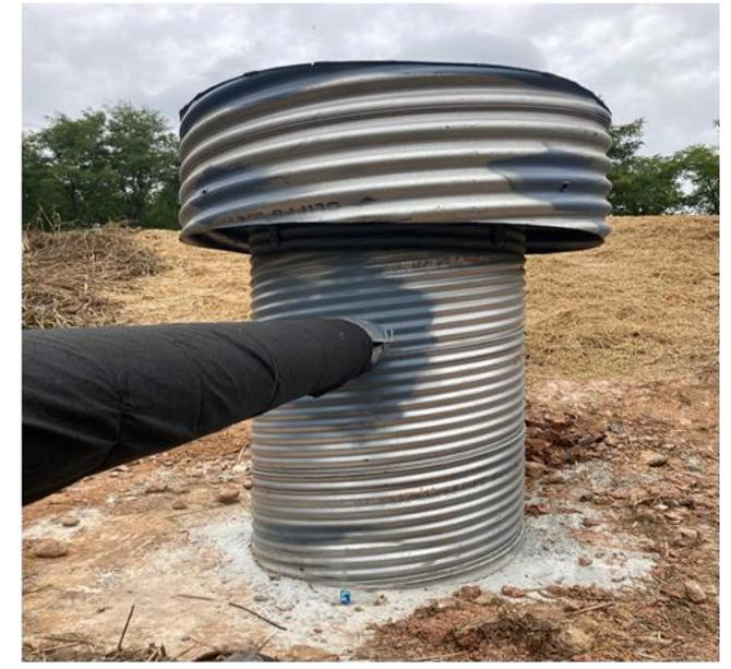
Riser replaced at Sediment basin 5 at Cell 6 North facing slope base.
