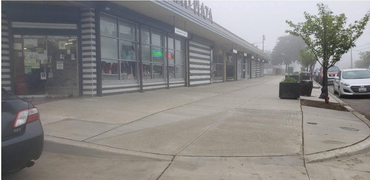
Sidewalk installation completed May 2019.
