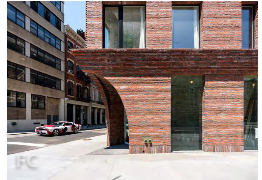
100 Franklin Street, NY
