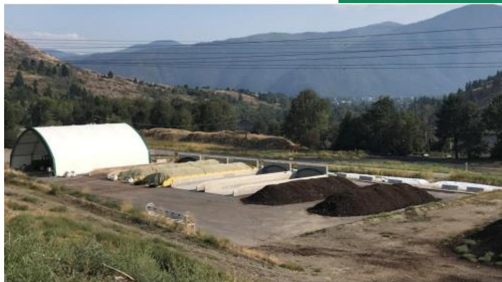
SG BUNKER® SYSTEM Grand Forks, BC, Canada
