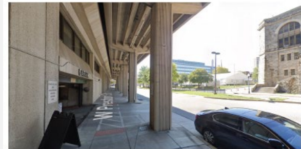
201 W Preston Garage ENTrance
