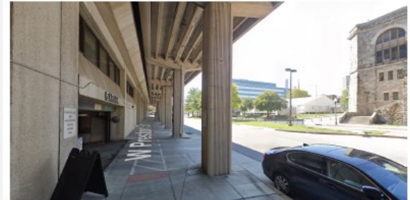
201 W Preston Garage Entrance
